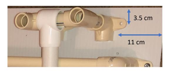
Measure 11 cm and 3.5 cm as shown in the picture. When you have the 3.5 cm, do a mark with a pencil. Put the elbow wing as in the picture, so you can do a mark in the other side of the elbow wing to drill. Drill and screw. Measure 1.5 cm from the screw, do the mark, review that you have 3.5 cm and drill. Put the elbow wing, do the mark, drill and screw.
